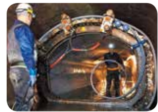
Rehabilitation of large diameter pipes (under construction)
