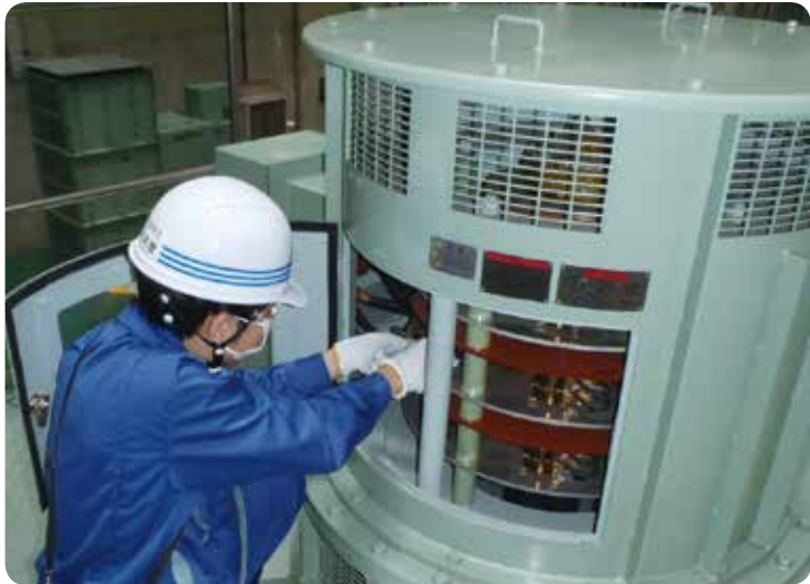
Inspection of high-voltage motors
