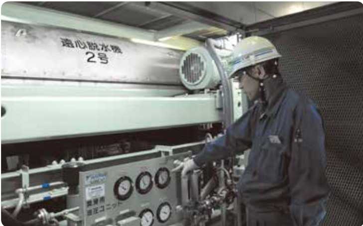
Inspection of dewatering facilities
