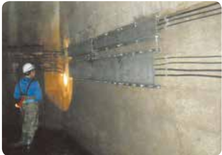
Inspection of optical fiber cables
