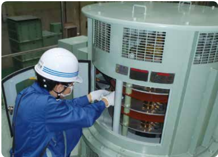
Inspection of high-voltage motors
